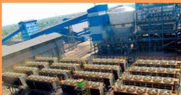
Adiabatic cooling towers at HZL-Dariba
